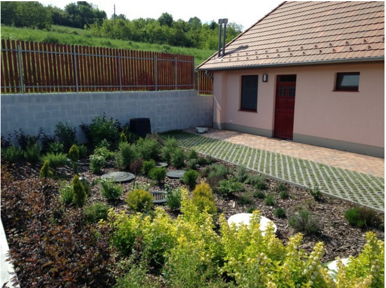
Picture 4: Waster water treatment and rainwater storage.
